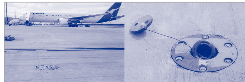
The Flush Mounted Anchor Point designed by Gilmore Engineers bolted into the tarmac at Brisbane International Airport prevents cargo planes from an unscheduled lift-off in high winds.
